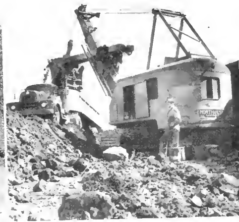
LEFT—Constructing embankment. RIGHT—Shovel excavating cut.
